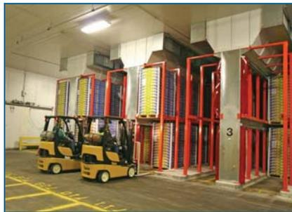
The Port's new Rapid Cooling chambers can cool up to 80 pallets from 40-45 °F to 32-34 °F in 3.5 hours
